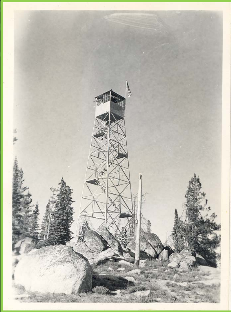
The only 7' x 7' Aermotor Co. steel cab lookout tower on the Boise NF
